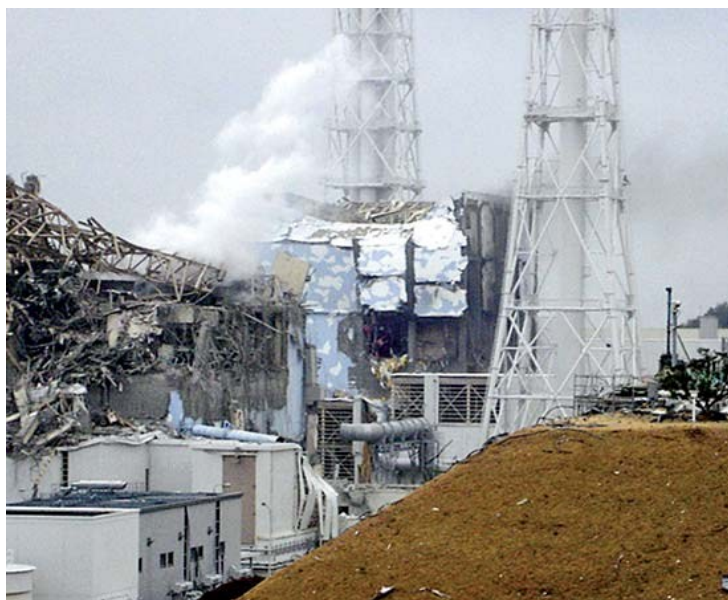
Two of the damaged containment buildings at the Fukushima Daiichi nuclear power plant, northeastern Fukushima prefecture, Japan, several days after the March 11, 2011, earthquake and tsunami that crippled the installation. Source: Tokyo Electric Power Co.—Kyodo News/AP
