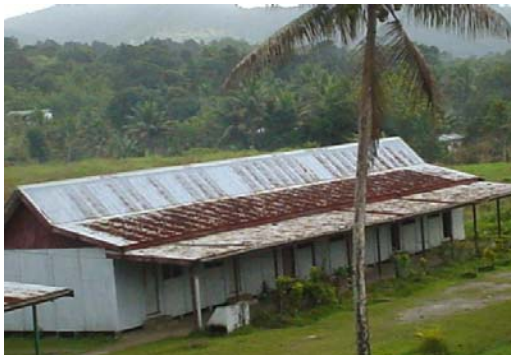
Lami High School: re-roofing done by Rotary Suva North.
